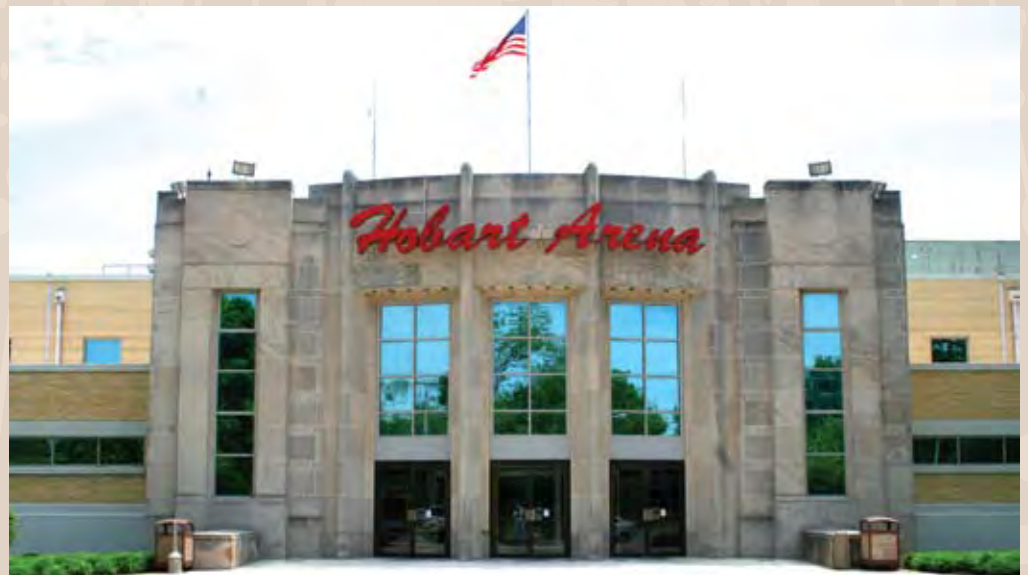
Photos on this page courtesy of André Odermatt and the Hobart Institute of Welding Technology
