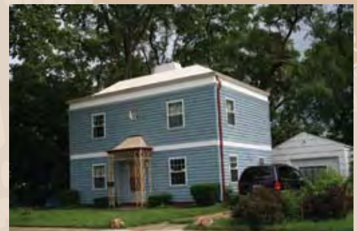
2-9 Hobart Circle Other Steel Houses
