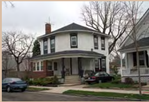
511 W. Race St., 1870 ▲ This house is one of a small number of octagon-shaped houses left in Ohio. Built about 1870 of poured gravel in cement, it was plastered and then stuccoed. It had French doors facing east and west and formerly was situated across the street from where D.A. Meeker (see page 37) lived. Pipes that were used for communication throughout the house and its odd shape caused children to call it “the haunted house.”
